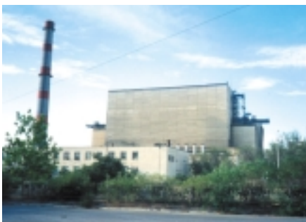
The BN-350 fast breeder reactor outside Aktau in western Kazakhstan is one of the sites where the United States has helped install advanced nuclear materials protection, control, and accounting (MPC&A) systems. The output power (350 MW) of the reactor is used to desalinate Caspian seawater for drinking and industrial purposes, to generate heat for commercial and residential use, and to generate electricity for the local area. The BN-350 achieved first criticality in 1973 and was operational until mid-1999.
